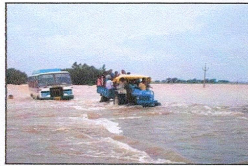
Fig-3: Road affected by flood
